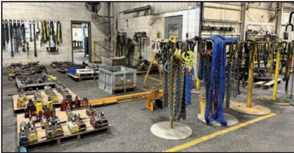
VIEW OF RIGGING
